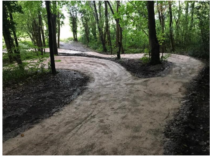
Figure 1.02: Beggar’s Bush Lane trail section after refurbishment in October 2019. (Pedal Progression, 2019)
